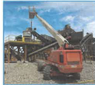
A miner fell 28 feet from an aerial lift basket. While he was wearing a fall protection harness it was not attached to the basket's anchor point.
